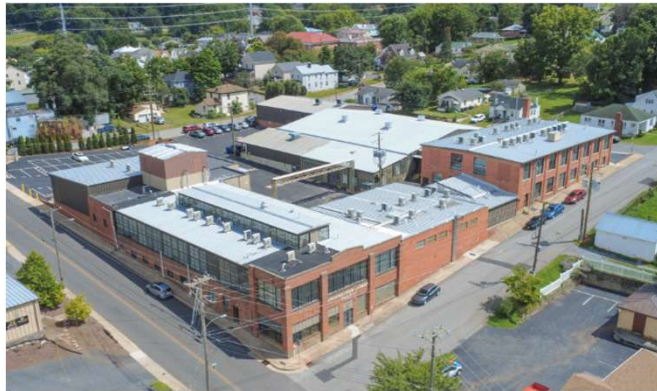
Staunton Steam Laundry Apartments
